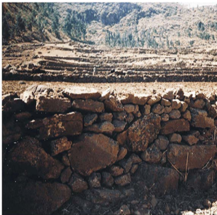
Fig. 6: Stone bund constructed in Afama Bancha Kebele (SNNPR, Ethiopia) Source: Melese [40]
