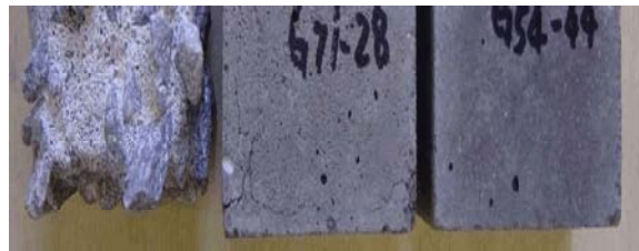
Fig. 2: Appearance of concrete specimens exposed in 10% sulphuric acid –Left Control Concrete for 28 days, right-Alkali activated concrete for 56 days (XJ Song)
