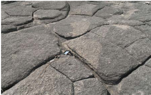
Fig. 5: Joints on Biotite Granite (Miango Complex)
