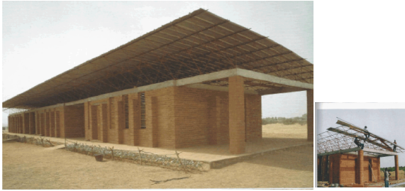
Plate 1: Primary School, Gando, Burkina Faso, 2001 [3].
