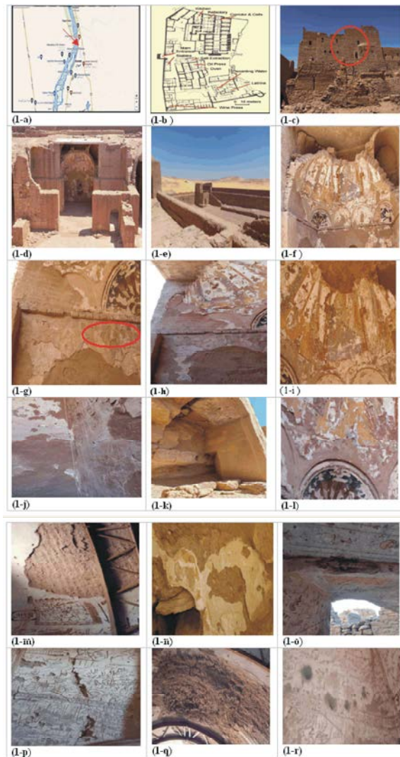
Fig. 1: (from a to r): Location and status of the Anba Hydra monastery. a: Map showing the location of the monastery of Anba Hydra. www.google.com/maps/ . b: shows the plan of the monastery. c: shows the construction of the Anba Hydra monastery on two levels. d : An overhead view of the church Ruins of a church on the lower level, with plaster and painting details. e: shows the desert surrounding the monastery. f: shows the vaulted arch and salts on the surface of the bricks in Al-Haniyah. Photograph taken in 2019. g : shows the remains of a painting of haloed figures seated and shows the loss of mortar. Photograph taken in 2019. h : showing the effect of wind on the main structure. Photograph taken in 2020. i: shows the color peeling, falling layers of plaster and the final disappearance of drawings from the vaulted arch and walls of the monastery. Photograph taken in 2019. j: shows the separation of the surface layer from the support. and damage from the Hajj's room k: shows the deep cracks caused by the loads at the inlet of the fryer. l: depicts a detail of the semidome and the separation of the colour crust due to temperature differences. Photograph taken in 2020. m: shows a fall in the plaster layers, which are to be completed from the inner walls of the room. We also see rust on the walls. n: Falling of plaster and cracks in building materials. o: Ceiling of cave at the west end. It served as an ancient Egyptian rock tomb that was used by monks. Paintings are dated to 600 or 700 AD. p: Murals and paintings in arched rooms beside the northeastern corner display the cracks resulting from the loads in the Anba p : Murals and paintings in arched rooms beside the northeastern corner display the cracks resulting from the loads in the Anba. q: shows the previous restoration on the walls while preserving the integrity of the wall below the beehive and not scratching the surface. r: Illustration of the concentration of fossilised hives on the walls.
