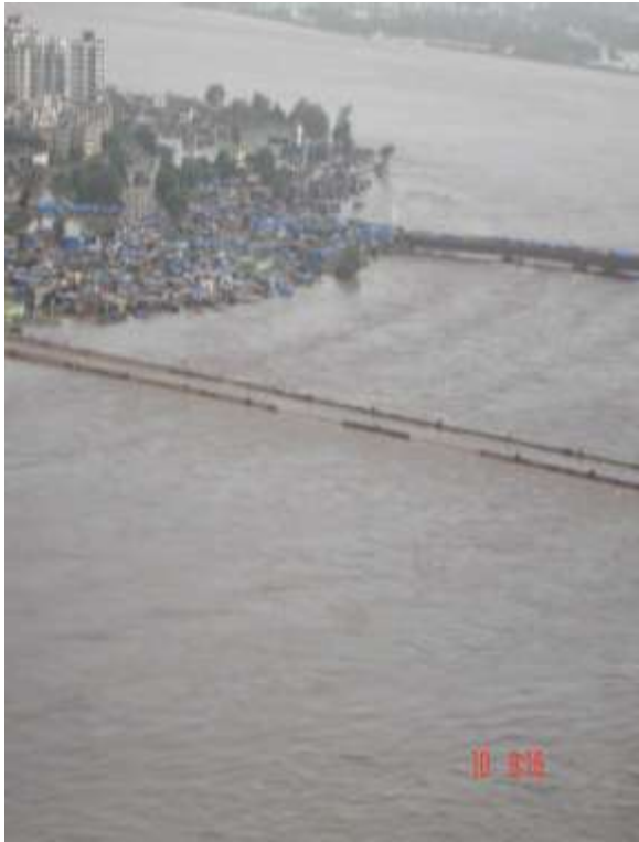
Fig. 4: Overflowing bridges during flood
