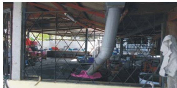
Pic. 2: Simple Rain Water Harvesting System in Sri Pulaui mosque. Skudai, Johor Baharu. Harvested Water Used Especially for Utensil Cleaning
