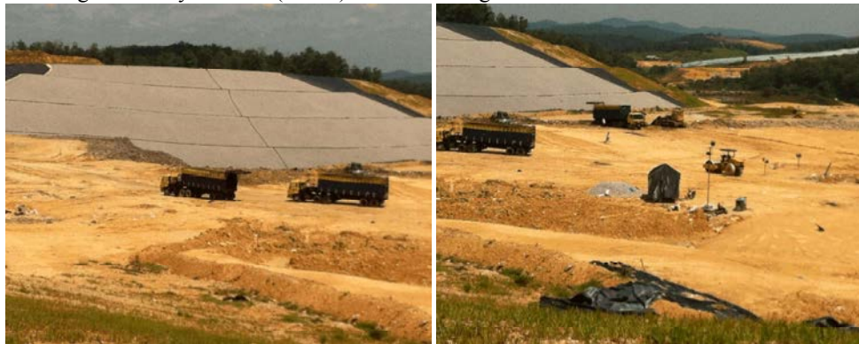
Fig. 5: High Density Polyethylene (HDPE) cover used at BTSL
