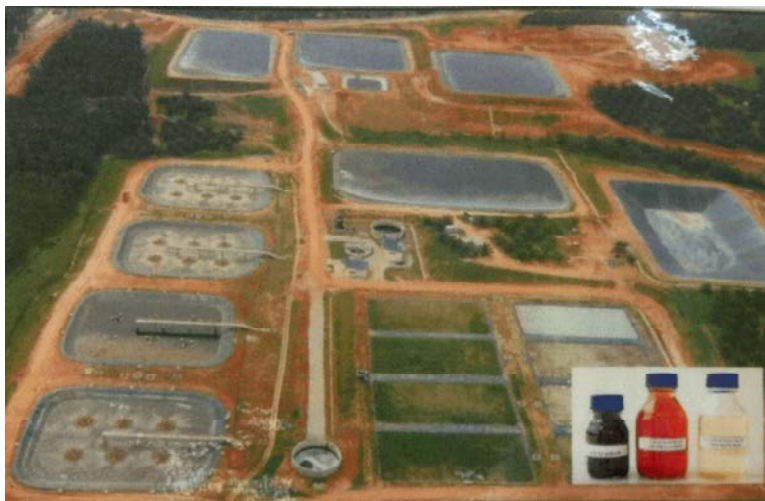
Fig. 6: Leachate treatment system at BTSL
