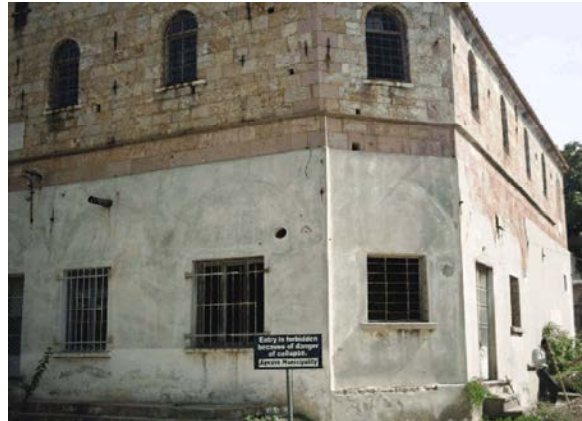
Fig. 1: Masonry walls in the lower floor formed later
