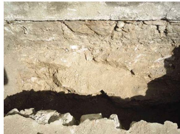
Fig. 2: Foundation of Stone Wall
