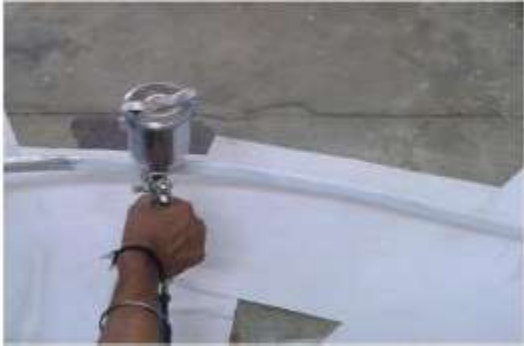
Fig. 12: Spray process on conductor with white emulsion
