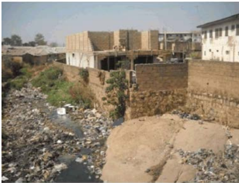
Fig. 4: Buildings within channel showing septic discharging into the river at GadaBiu
