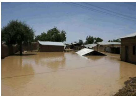
Fig. 8: Flood around the study area: Source NEMA 2012
