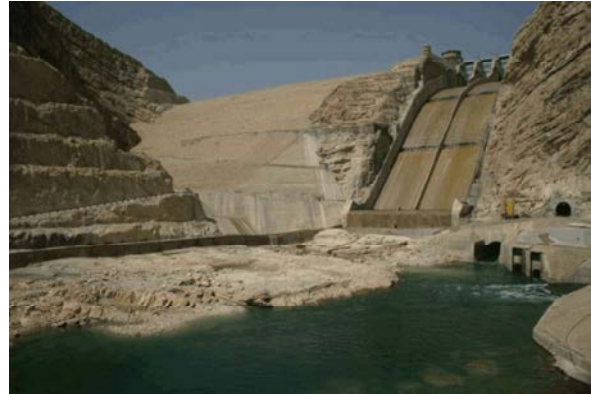
Fig. 1: View of dam-Behbahan, Iran
