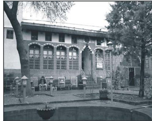
Fig. 8: View of winter room from the courtyard
