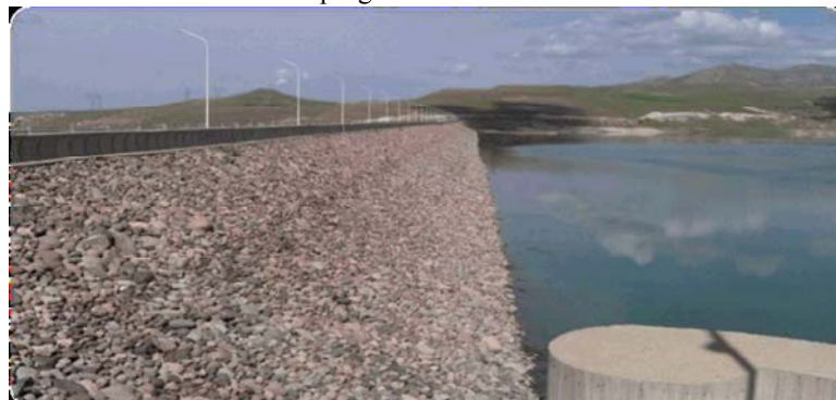
Fig. 1: Upstream slope of Alavian reservoir dam
