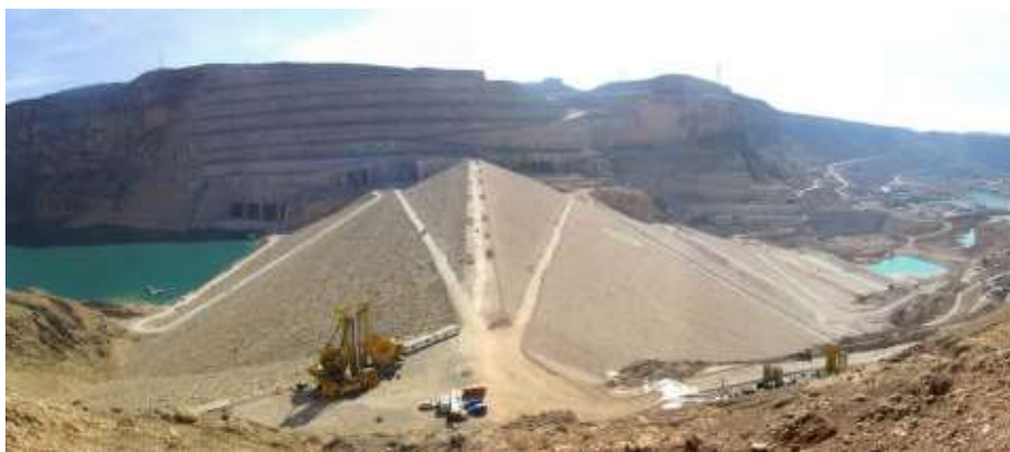
Fig. 1: Landscape of top crest of Gotvand-Olya Dam
