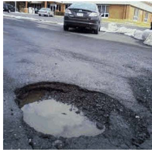
Fig. 1: Condition of roads with potholes
